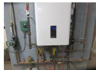
The bottom right photo shows the replaced piping and the white gas-fired heat/hot water unit. It too required maintenance. The tankless hot water system delivers hot water much more quickly now!
